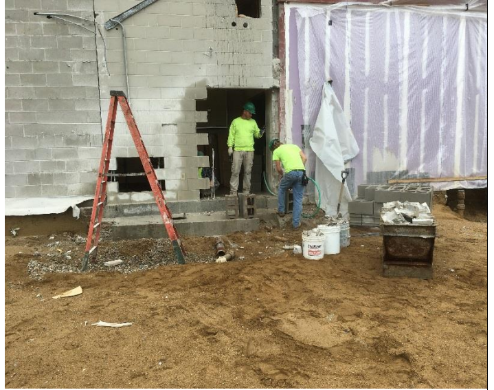
Masonry Infill @ New Kitchen Area 10-03-18
