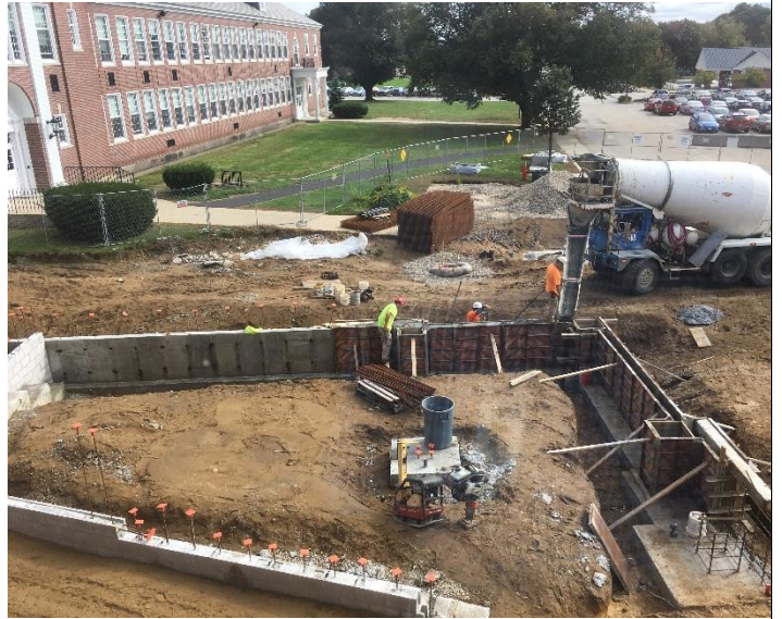
Foundation Concrete Placement @ CL 22 & K.1 10-03-18
