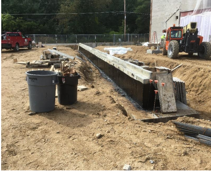
Foundation Waterproofing @ CL 20 10-03-18 (1)
