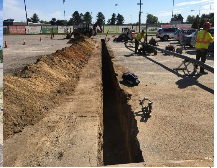
Unitil Gas Line Expansion @ Student Parking Area 7-10-18 (2)
