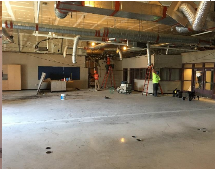
Phase-1 Concrete Block Demo Rm's 210-220 7-10-18 (2)
