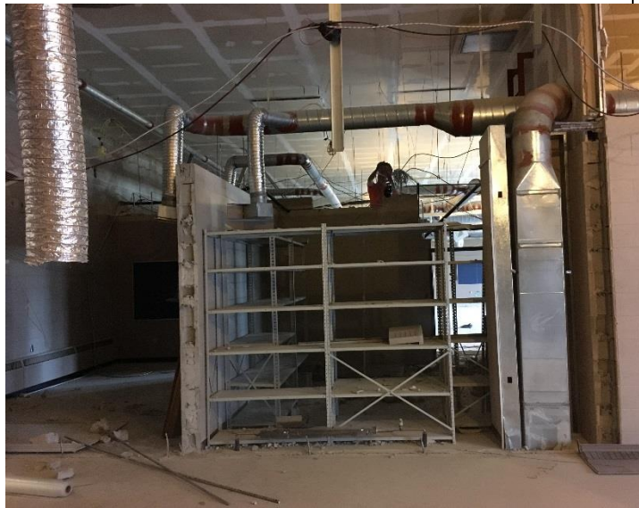
Phase-1 Concrete Block Demo Rm's 210-220 7-10-18 (1)
