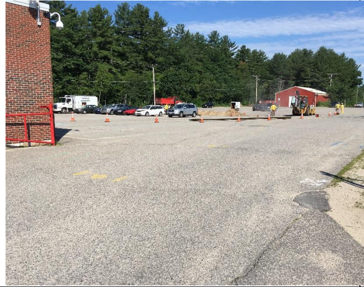
Unitil Gas Line Expansion @ Student Parking Area 7-10-18 (1)
