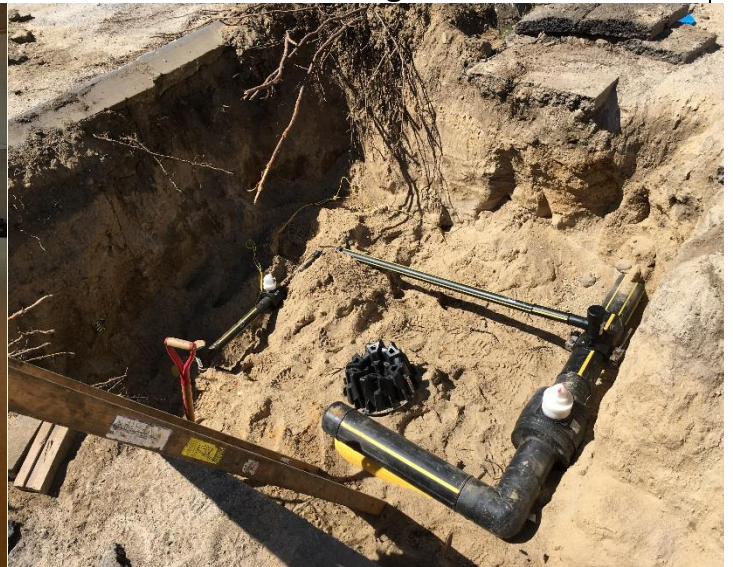
Unitil Gas Line Expansion Bypass Pipe & Valves @ Student Parking Area 7-12-18
