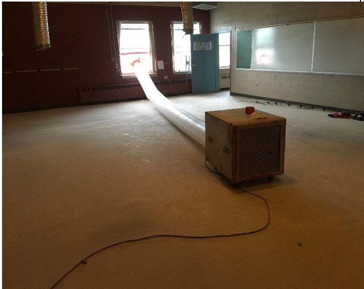
2nd Fl. Operating Negative Air Exhaust Unit 7-11-18
