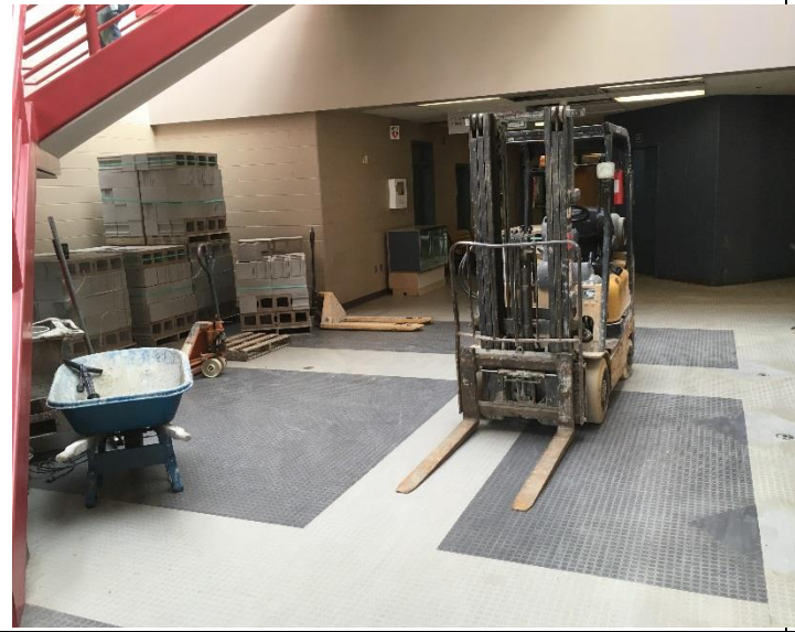
Shear Wall Block & Lift 7-17-18 (1)
