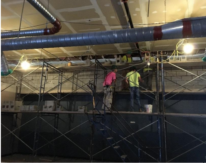
Rm. 210 Shear Wall Staged Block 7-18-18
