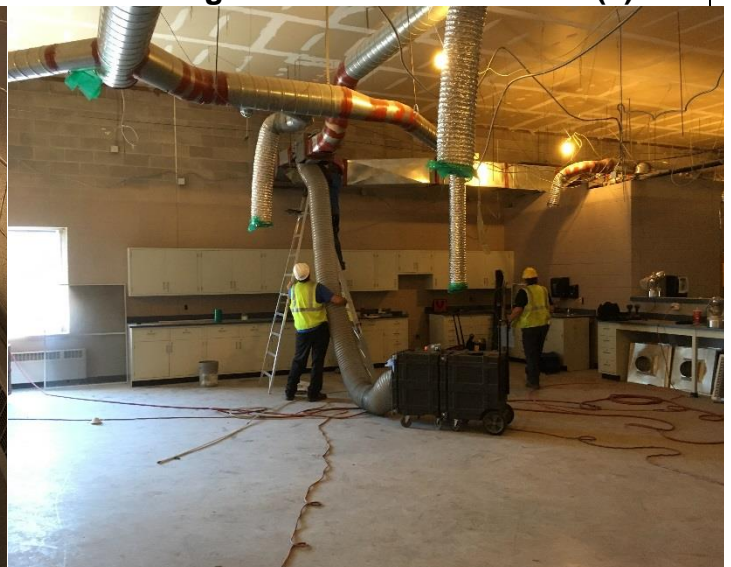
Duct Cleaning Phase-1 2nd Fl. 7-18-18 (2)
