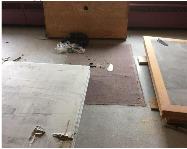
Rm.220 Floor Below Removed Built-In Table 7-11-18 (1)
