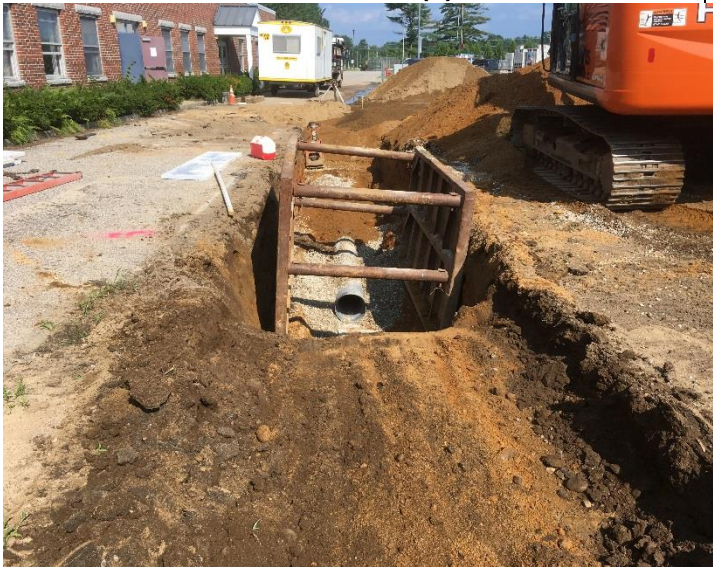
Storm Drain Pipe From Existing CB To New Drain Manhole DM-20 8-16-18 (1)
