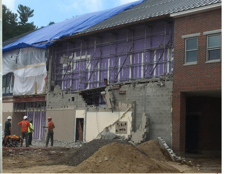
Main Entrance Demolition 8-16-18
