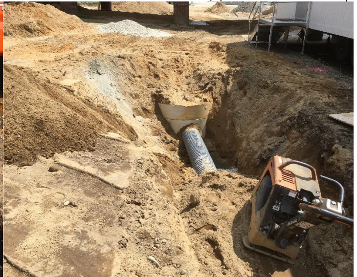
Storm Drain Pipe From Existing CB To New Drain Manhole DM-20 8-16-18 (2)
