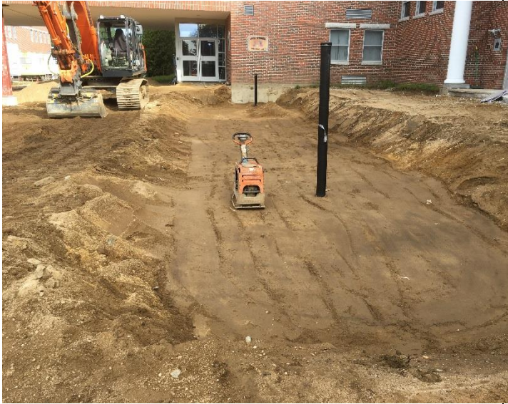
Backfill & Compaction Over New Roof Drain Piping 8-23-18 (1)
