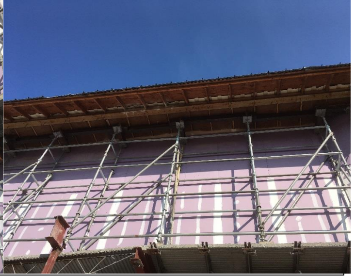
Shoring Scaffold Supporting S Elev. Of Existing Building 8-27-18 (3)
