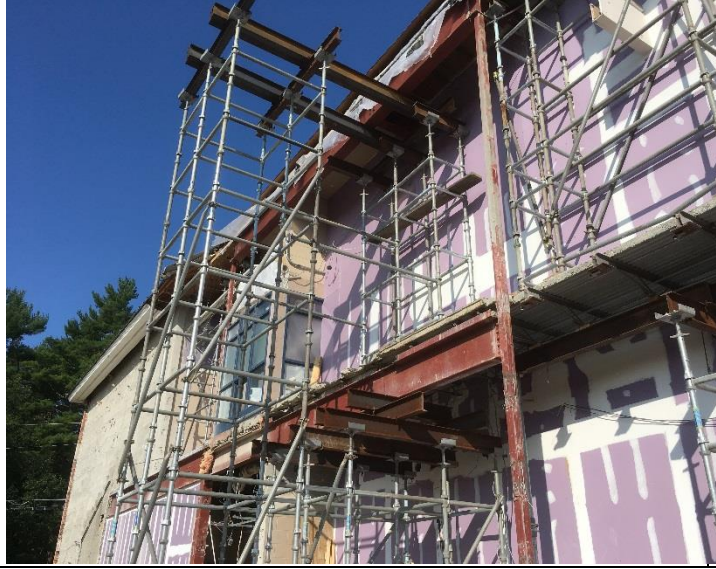
Shoring Scaffold Supporting S Elev. Of Existing Building 8-27-18 (2)
