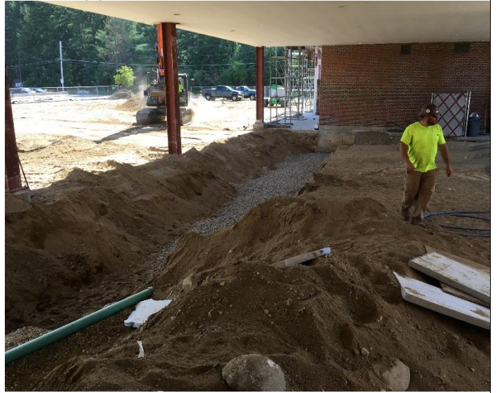
Stone Base For Concrete Footings Below Bridge 9-04-18 (2)
