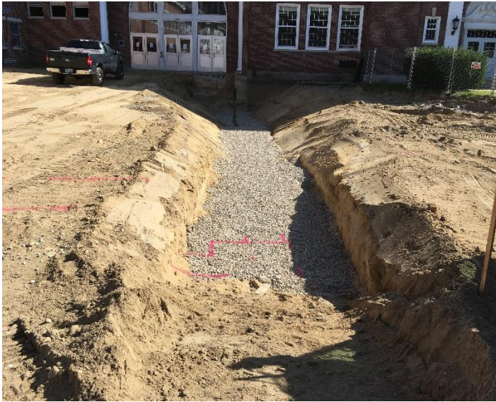
Stone Base For Concrete Footings 9-04-18
