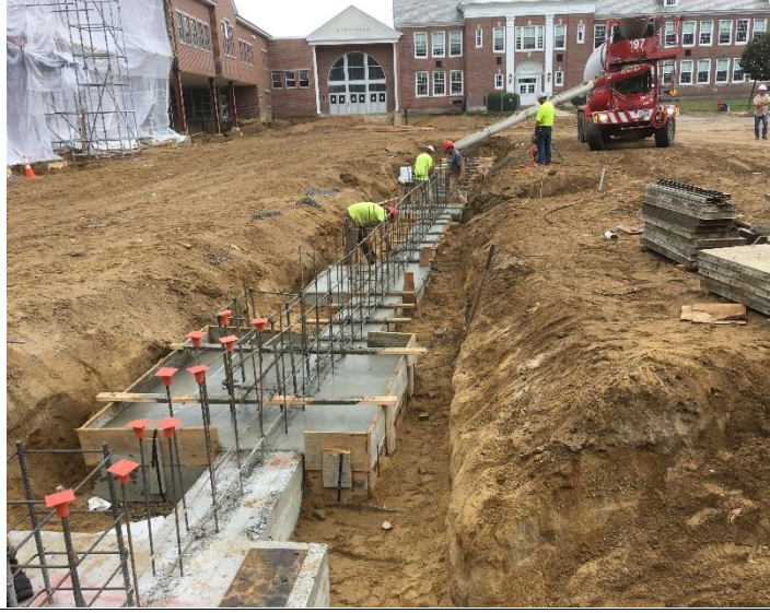
Concrete For Footings @ CL-20 9-12-18 (1)
