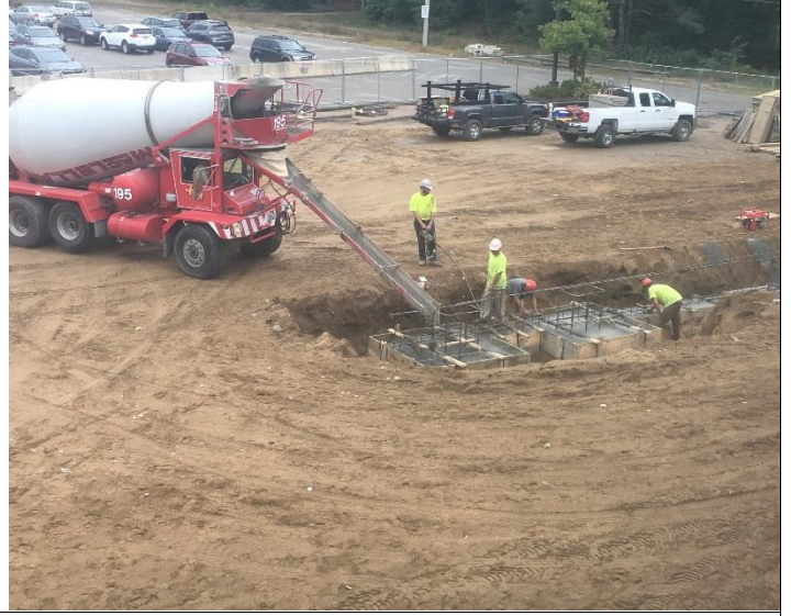
Concrete For Footings @ CL-20 9-12-18 (2)
