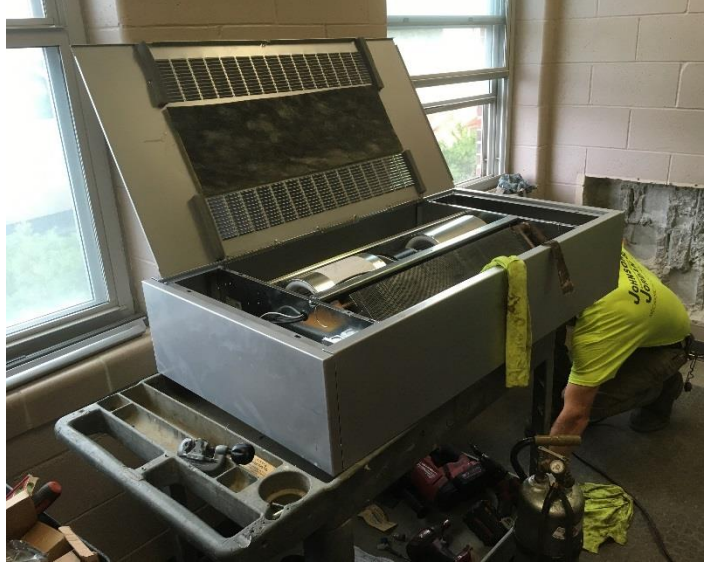
New Cabinet Unit Heater @ Stair-3 9-20-18 (1)
