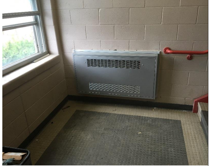
New Cabinet Unit Heater @ Stair-3 9-20-18 (2)
