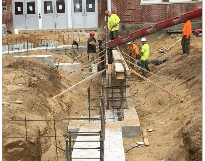
Excavation & Stone For Pier Footings 9-20-18 (1)
