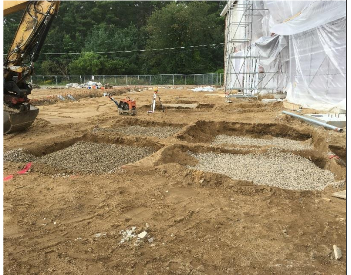
Excavation & Stone For Pier Footings 9-20-18 (1)
