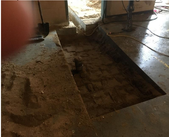
Compacted Backfill @ Rm's. 127 E-F 9-26-18 (1)
