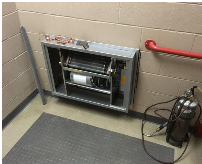
New Cabinet Unit Heater @ Stair-2 9-26-18 (1)
