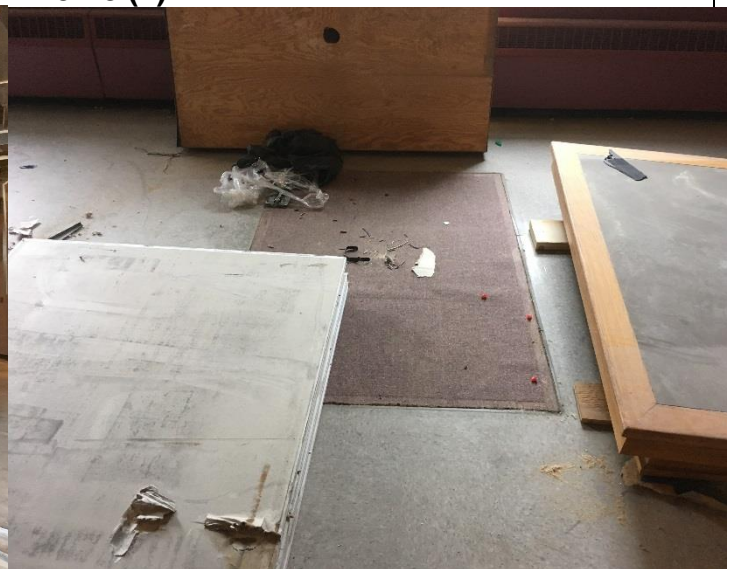
Rm.203 Floor Below Removed Built-In Table 7-23-18 (1)
